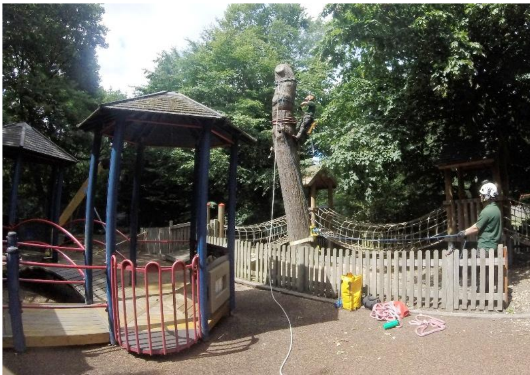
Figure 3: dismantling dead oak in play area
